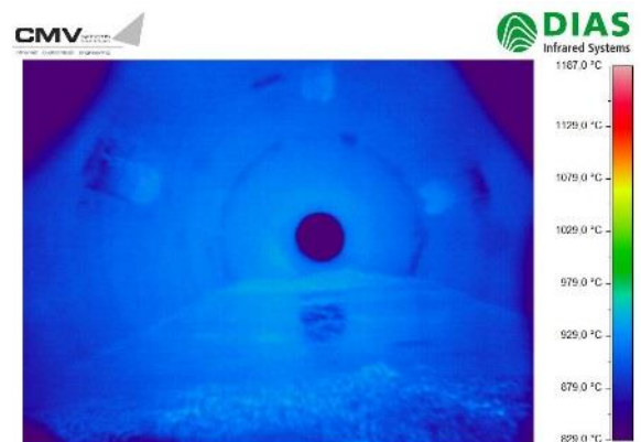
Infrared Image at the end of the process: Good visibility through the furnace in spite of high dust content.
