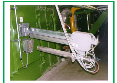
TV-INC TV-system for control of the burn out grate zone
