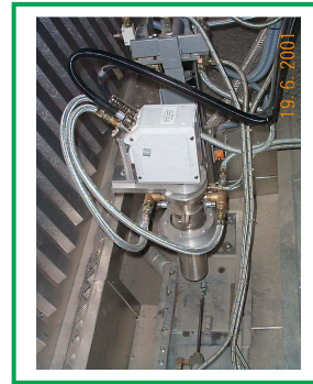
PYROINC256-IR-camera system for control the drying and combustion grate zone
